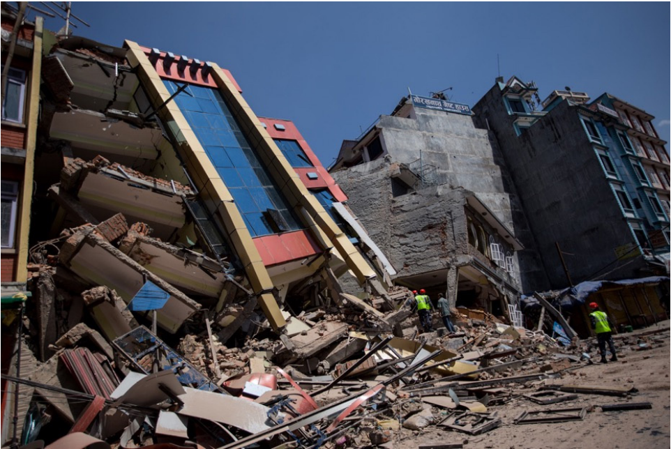
Earthquake aftermath, Kathmandu, Nepal, 12 May 2015
