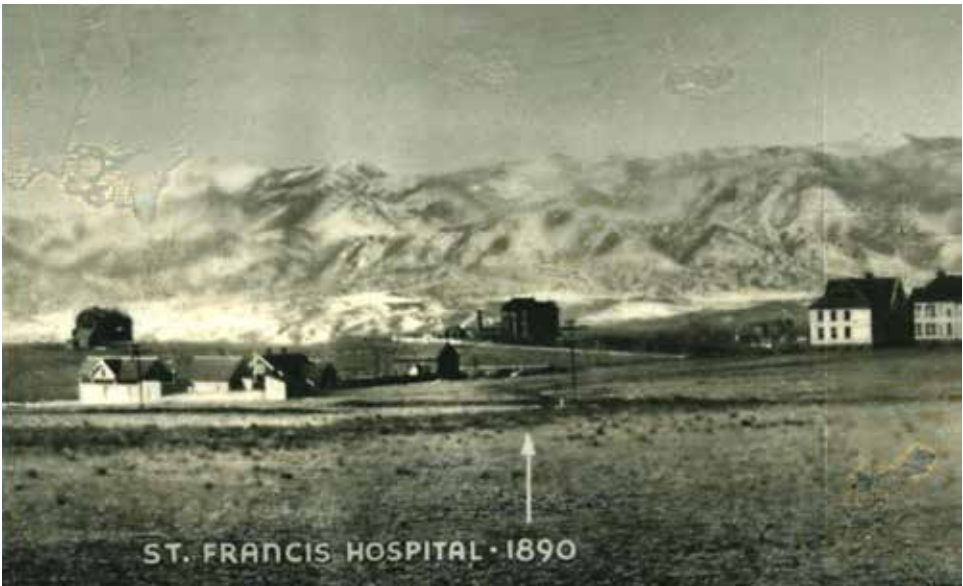
Original St. Francis Hospital of Colorado Springs, c.1890
